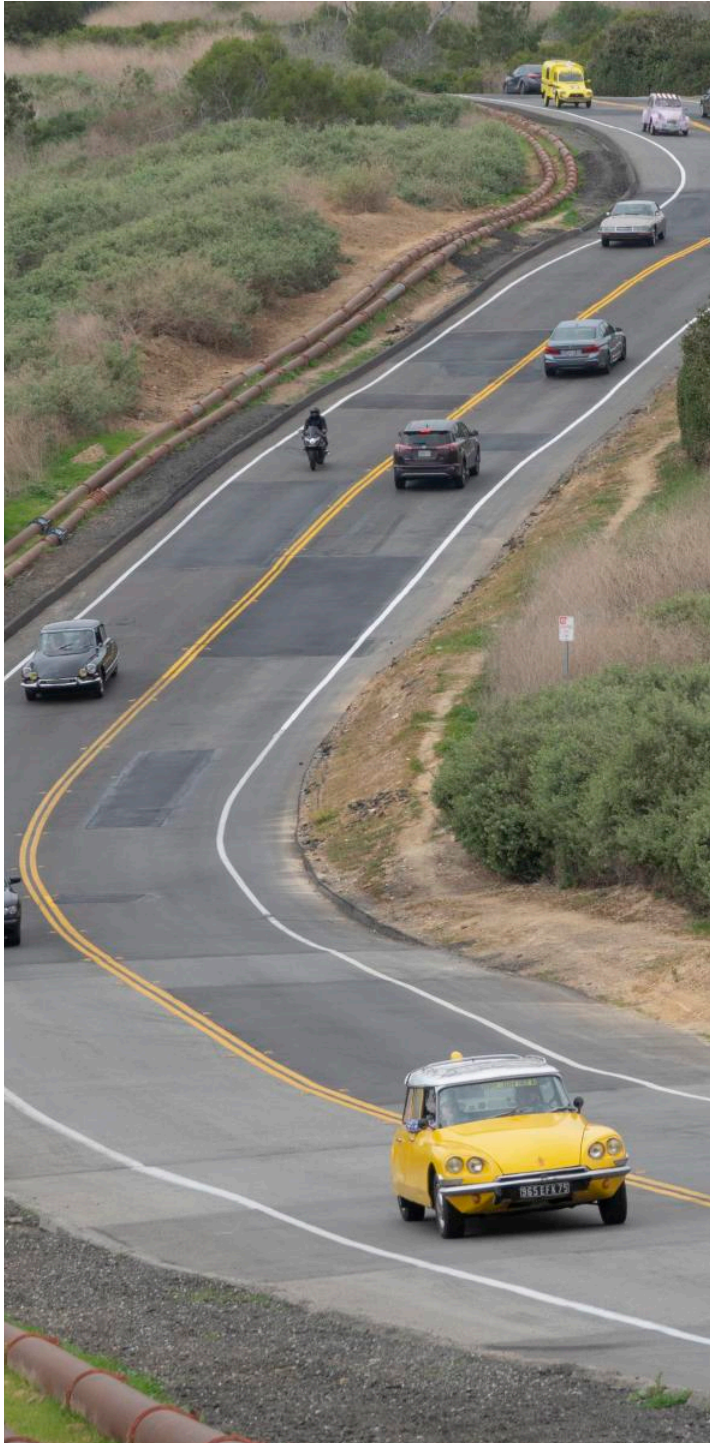
Above: PV Drive South at Portuguese Bend. The unstable land is shown in the wavy, off-patched paving and above ground plumbing.
